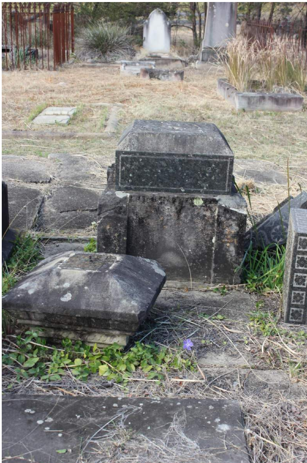
Figure 6: These pieces of a polished granite memorial have fallen from a monument. Given their weight, they could probably be retained on site but a search should be made for any other pieces, either of the column or of a surmount such as a sculpture. All pieces should be photographed and tagged—aluminium plant tags are obtainable from garden centres are useful for this purpose and can be written on with a permanent marker. Repair of this type of monument will probably require the use of phosphor bronze or high-grade stainless steel pins and appropriate adhesives to join the broken pieces. (Source: GML Heritage, 2014)
