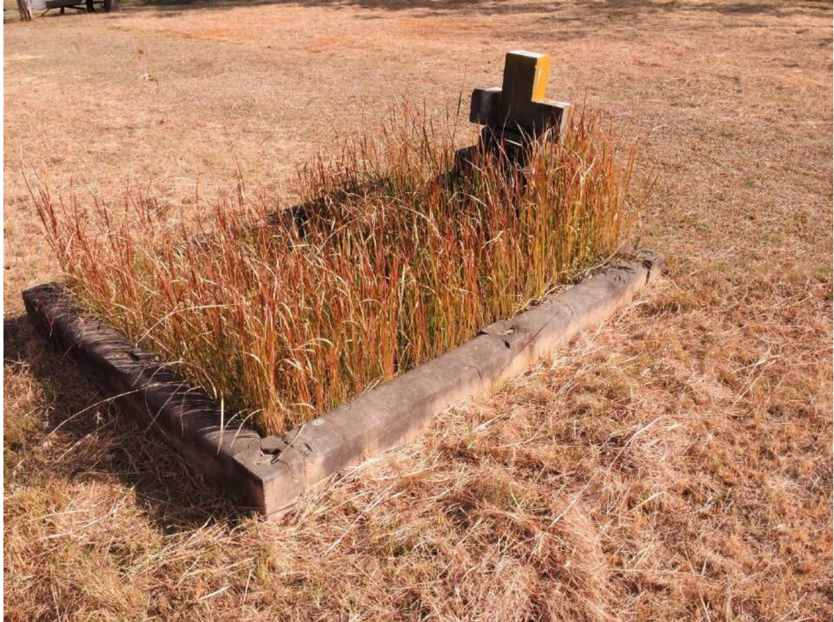
Figure 8: This grave is relatively intact, with its kerb in place and cross still standing. Dense grass growth obscures the surface of the grave which may be a tiled slab or a slab covered with marble or other chips. Retention of herbaceous material such as native grasses within kerbs is acceptable provided it does not exacerbate physical damage to the monument. Plant growth should be trimmed so that inscriptions can be read. (Source: Chris Betteridge, 2014)
