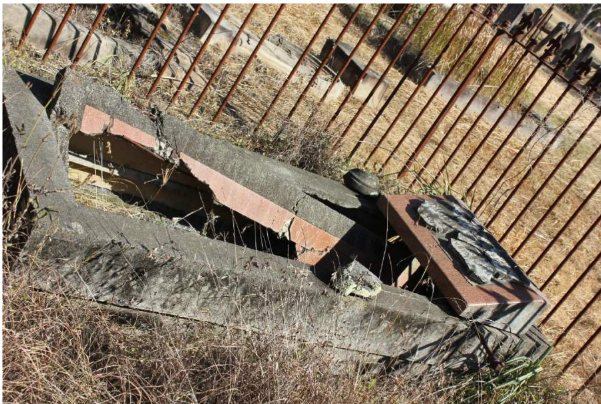
Figure 9: This desk and slab memorial has suffered considerable damage including breakage of the slab and dislocation of the desk, both of which feature ceramic tile upper surfaces. A search of the surrounding area should be made to locate the missing tiles which should be retained within the grave surrounds. Matching these tiles would probably be difficult but the original monumental masonry company may have a record of the source. Full repair of this memorial is probably not cost-effective but the grave could be improved by repositioning the desk to its original location and placement of the slab back inside the kerbs. (Source: GML Heritage, 2014)
