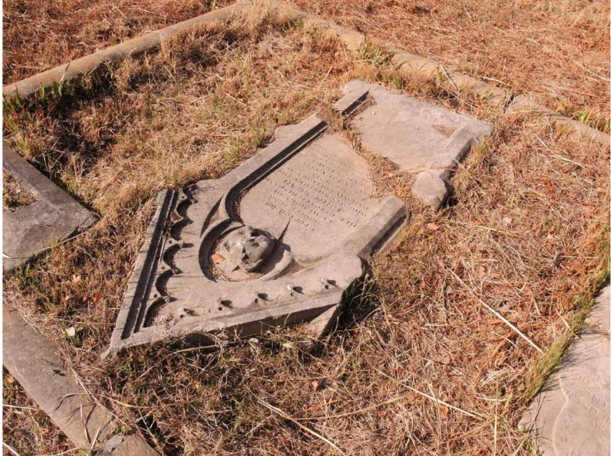
Figure 5: This stele has fallen and broken into two pieces. If it cannot be repaired and re-erected, it should be well supported and raised off the ground at the top so that water runs off the inscribed face. (Source: Chris Betteridge, 2014)
