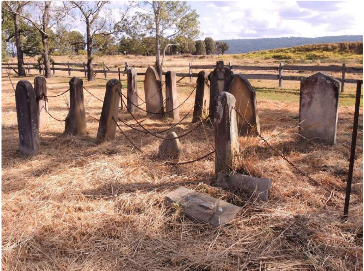
Figure 4: Plot with multiple grave markers with surround of chains attached to sandstone posts. Tilted or fallen posts should be righted and the chain preserved with fish oil. (Source: Chris Betteridge, 2014)
